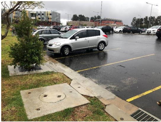
Figure 3: Example photos of the Filterra® biofiltration system and sampling facilities at the site
