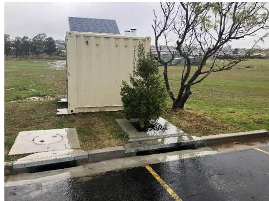
Figure 3: Example photos of the Filterra® biofiltration system and sampling facilities at the site
