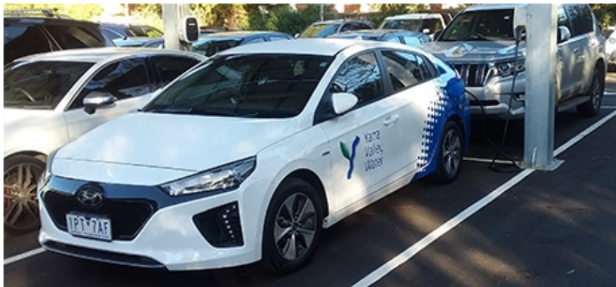
Figure 4: Fully electric vehicle being charged from the solar carport at Yarra Valley Water's head office
