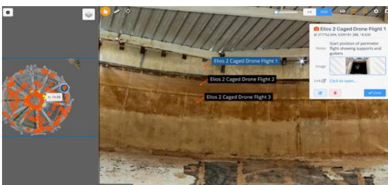
Figure 11 – Defect identification on the internal of the tank
